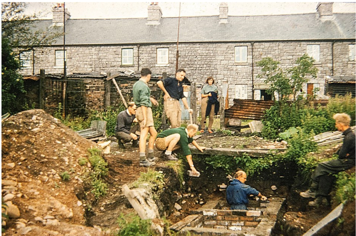
Constructing the septic tank, summer 1959.
