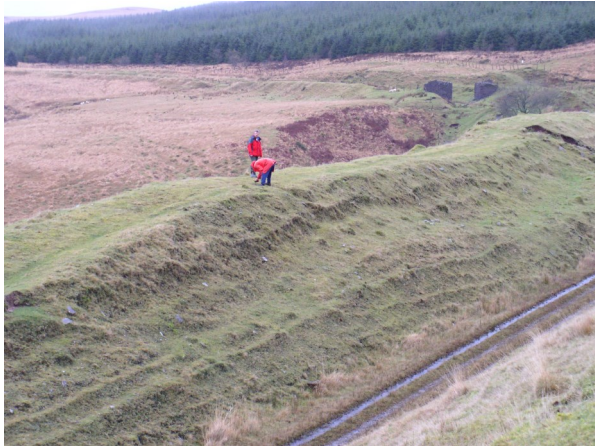
Above Left: Washout on the railway embankment.
